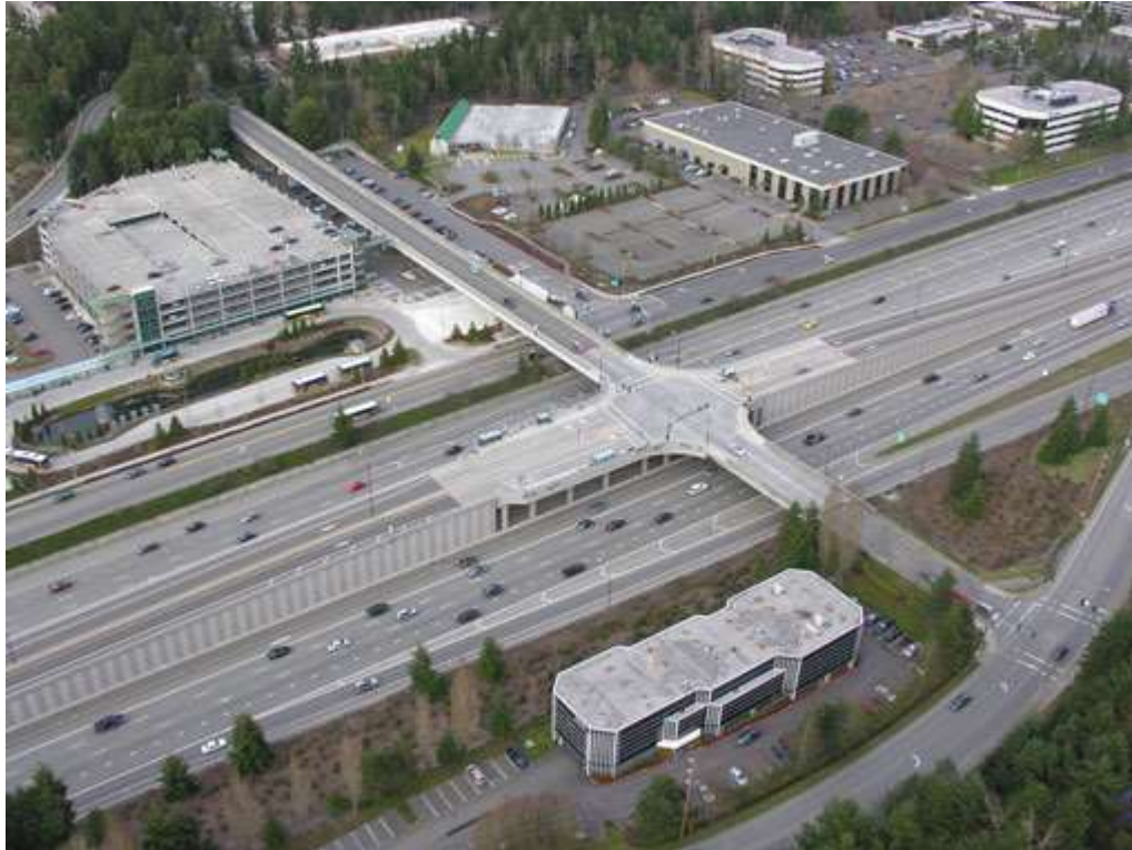
Fig. 9 Ramp system in I-90 in Seattle
