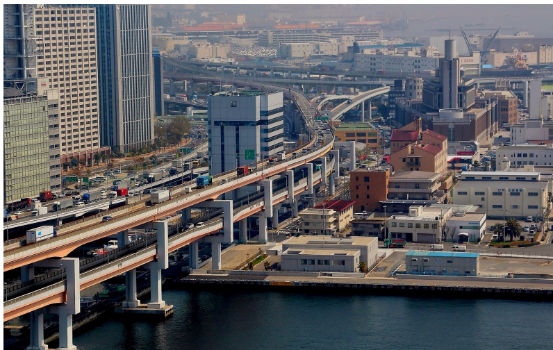
Fig. (1). Second floor of roads in Kobe, Japan.
